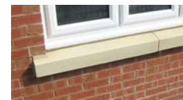
Cast stone cills and lintels
